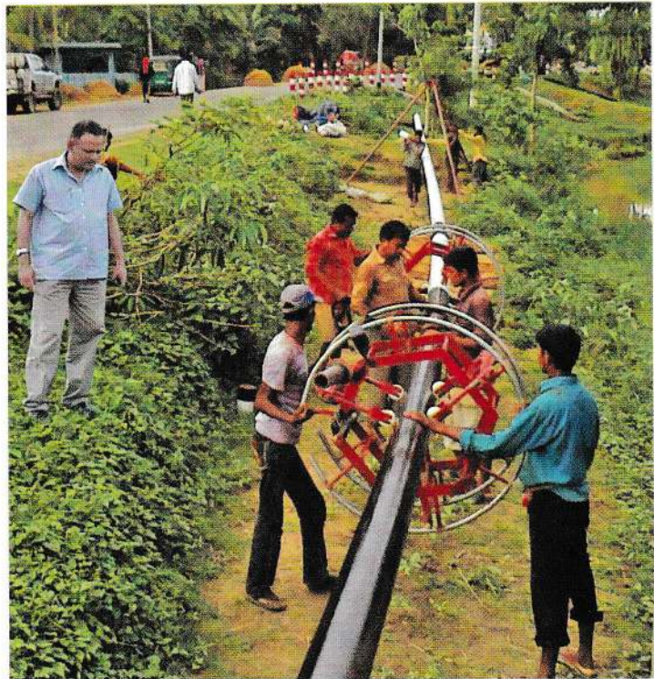
Pipeline construction works under Sylhet Gas Transmission Network Up-gradation Project
